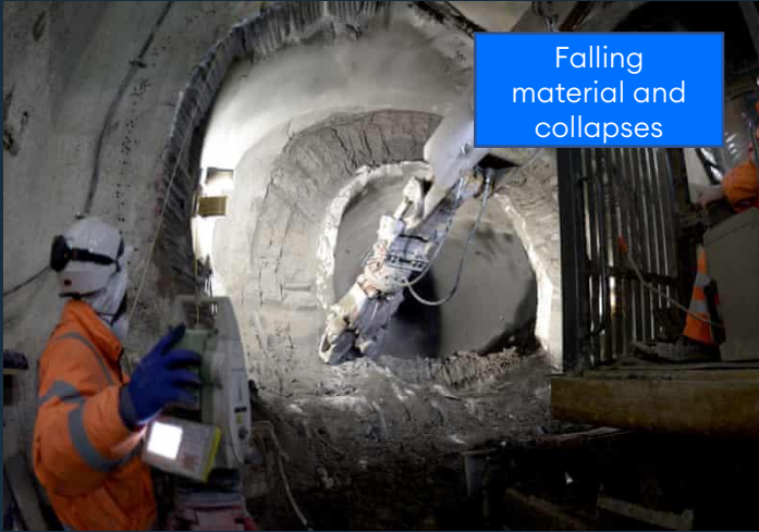
Red Zone within works areas in tunnels Preventing being injured through structure collapsing
