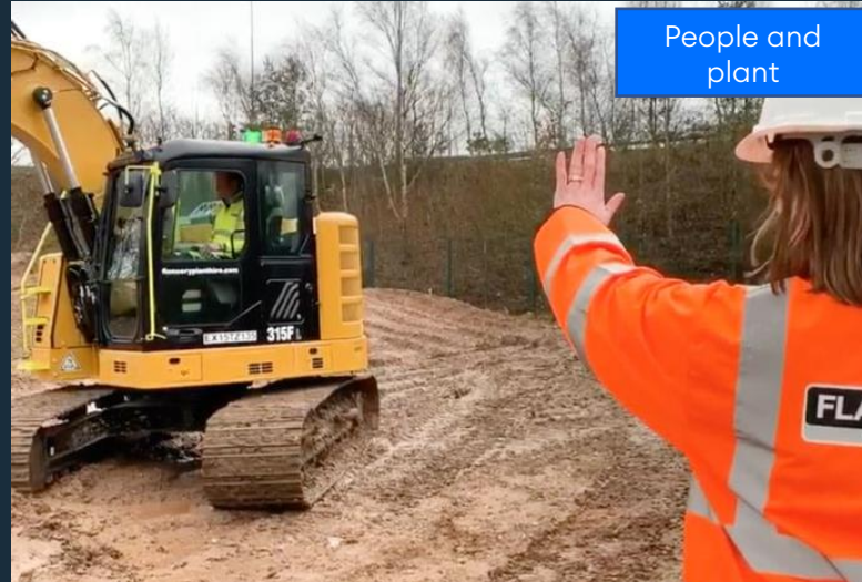
Red zone access around machinery Preventing people being struck by moving vehicles
