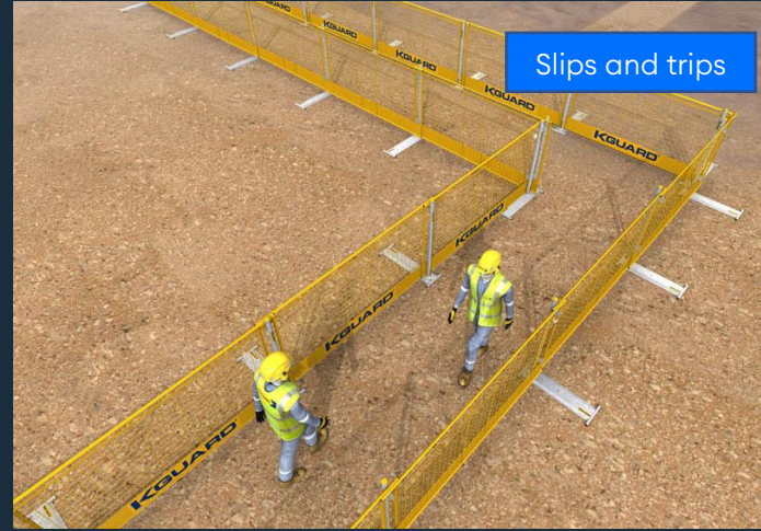
Red Zone outside accessway Preventing slips, trips and falls outside of designated clearways
