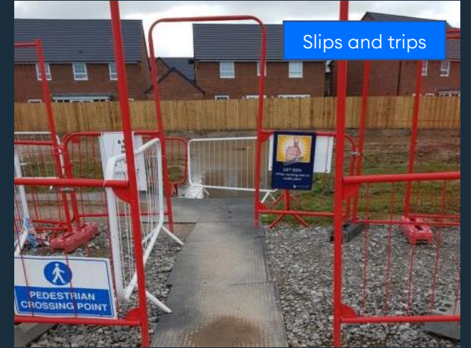
Red Zone outside accessway Preventing operatives being struck by moving vehicles outside of designated crossings
