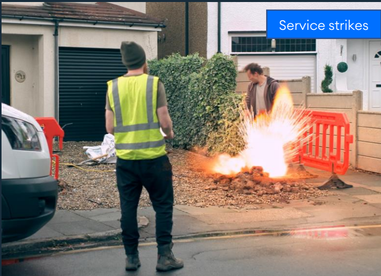
Control of tool use over the top of buried services Preventing electrocution / explosion and related cost impacts.
