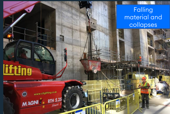
Red Zone inside lifting zone Preventing injury through falling objects/entrapment
