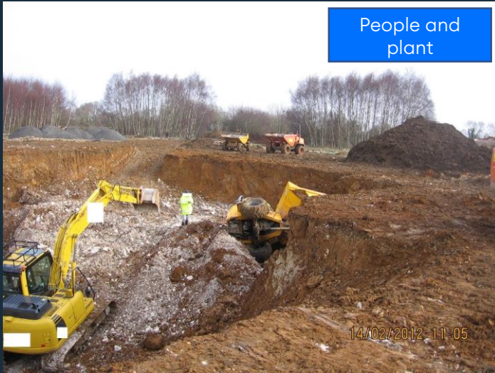
Red Zone around embankments Preventing being struck by overturning vehicles related cost impacts.
