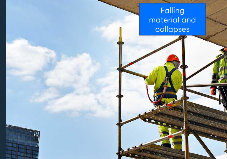
Amber zone access under overhead working area Preventing injury through falling objects
