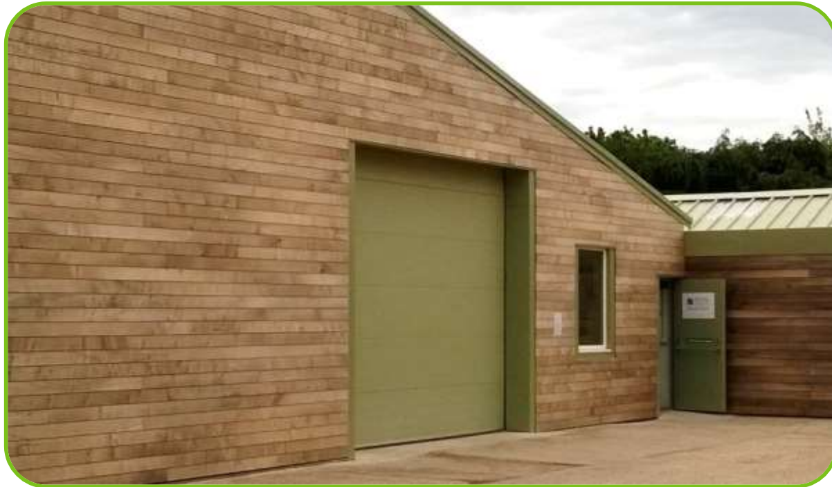
Brimstone Cladding, Sylva Wood Centre - Photo: SusConSol
